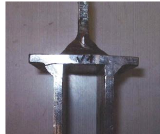
Figure 11: Crack along the weld leg section
